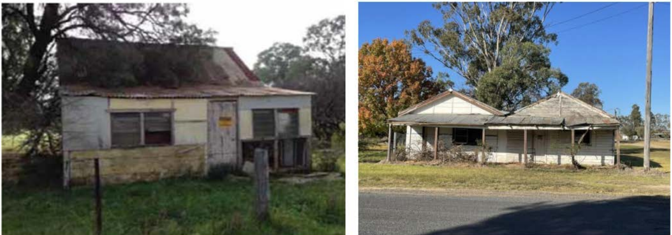
Figure 3 | Examples of WCPL owned structures in SIMP demolition program (Source: Modification Report)
